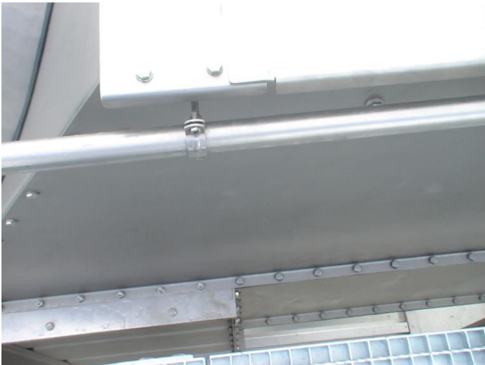
Figure 1.12 — Noise Source 12: Pipe anchor. Fix: Secure to flat surface.
