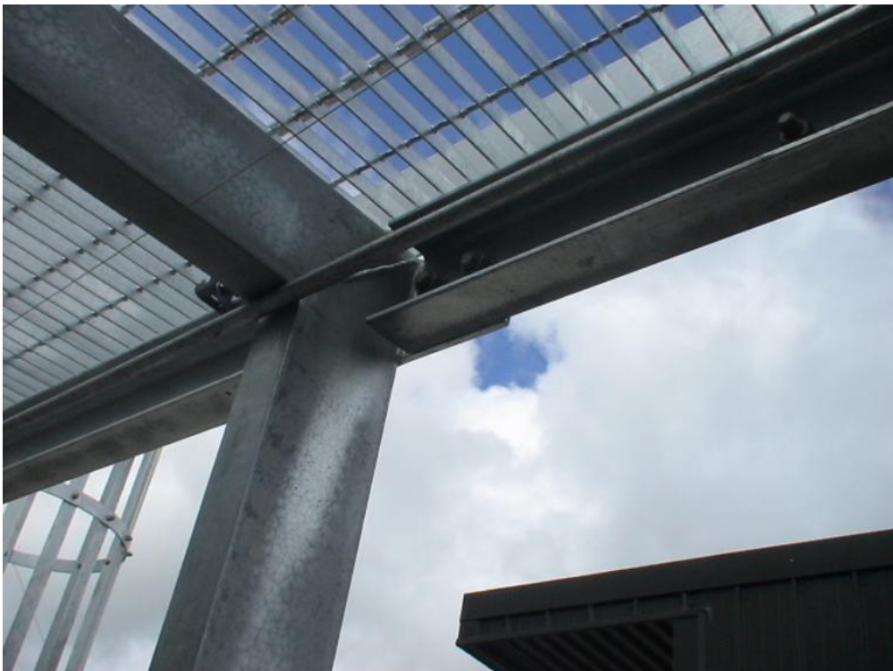
Figure 1.6 — Noise Source 06: Steel grating. Fix: Fill grating voids.
