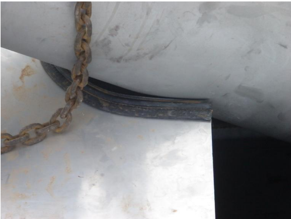
Figure 1.14 — Result after all fixes applied.
